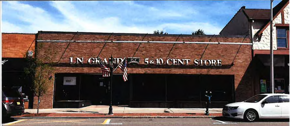
2. View of rear façade looking north.
